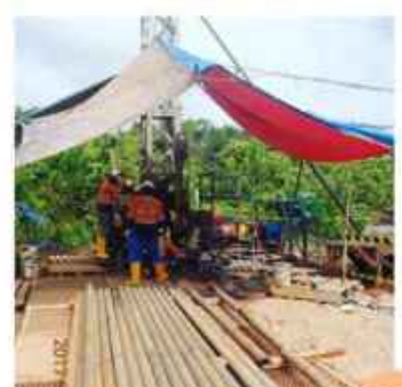
ARUTMIN INDONESIA COAL DRILLING
