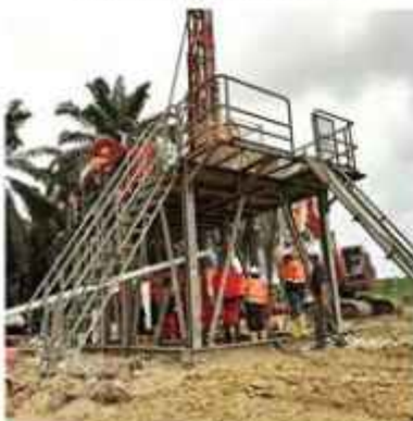
INDON CBM PTY LTD. CBM DRILLING
