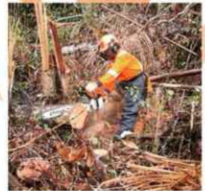
BHP BILLITON ACCESS PREPARATION
